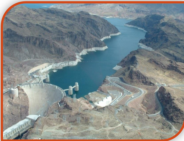
Hoover Dam, once known as Boulder Dam, is a concrete arch-gravity dam in the Black Canyon of the Colorado River, on the border between the US states of Arizona and Nevada. It was constructed between 1931 and 1936.
